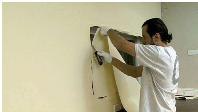
Cut open the window space.
