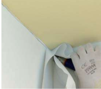
For corners, use a utility knife to remove the rest of the covering.
