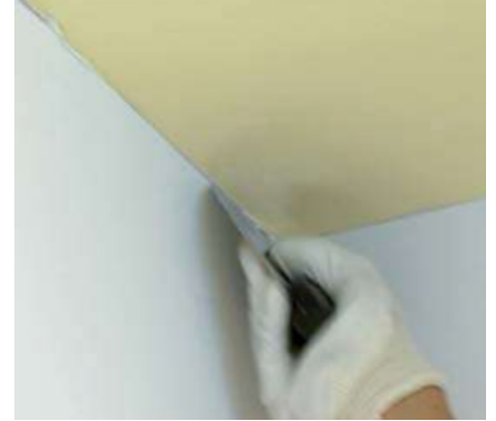
Press the covering's excess margin into the recess in the profile.
