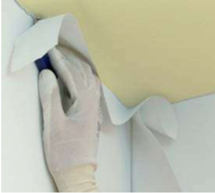
Trim the covering over the entire length using a utility knife.
